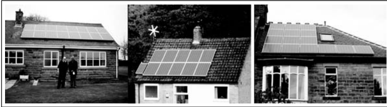
Figure 10.12 Solar roofs installed in Sheffield after the introduction of new solar tariff in the United Kingdom in April 2010. See also Colour Insert.
